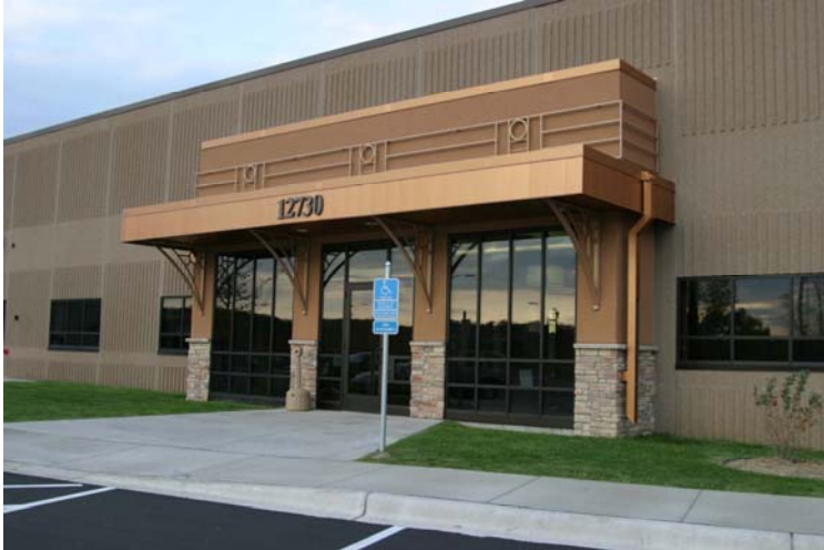
Datakey Electronics new facility at 12730 Creek View Avenue, Savage, MN 55378-2618.
